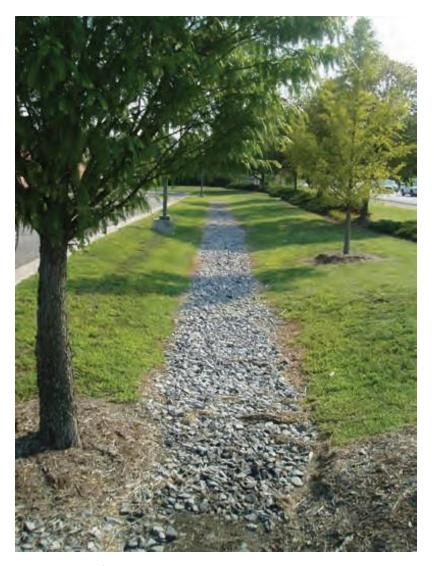
Figure 4.16. Infiltration practice in median strip.
