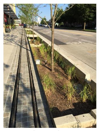
Figure 4.5. Example streetscape bioretention.
