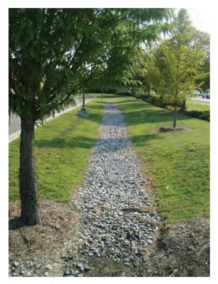
Figure 4.16. Infiltration practice in median strip.
